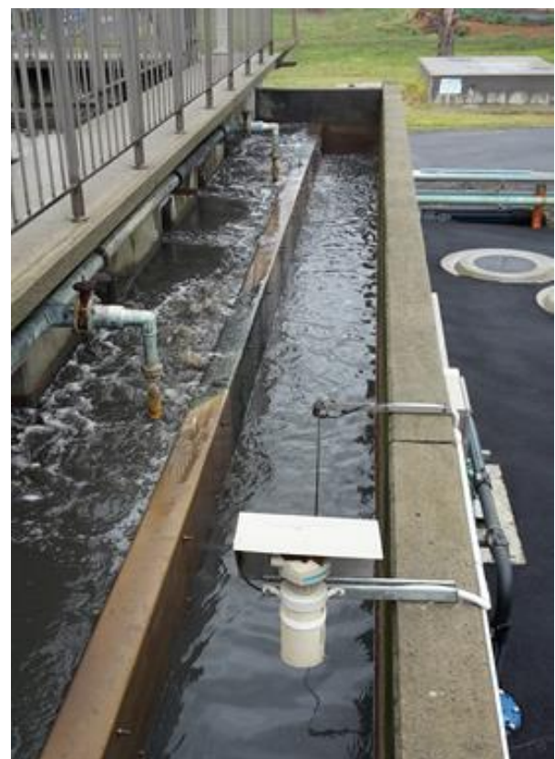
Bypass at Ti Tree Bend
