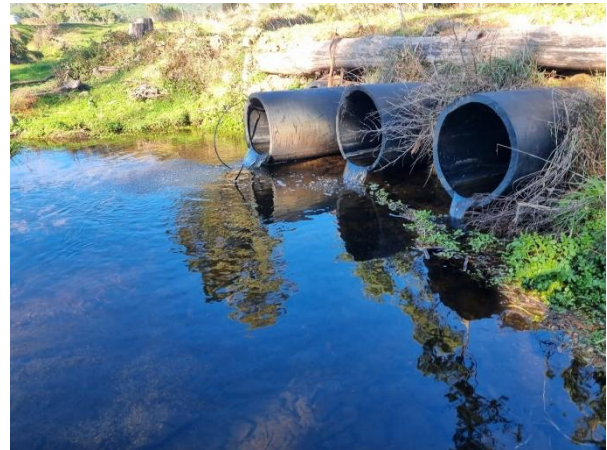
Giant freshwater crayfish are unable to even attempt passage through culverts that are “perched” above the water surface. Image credit: Todd Walsh.
