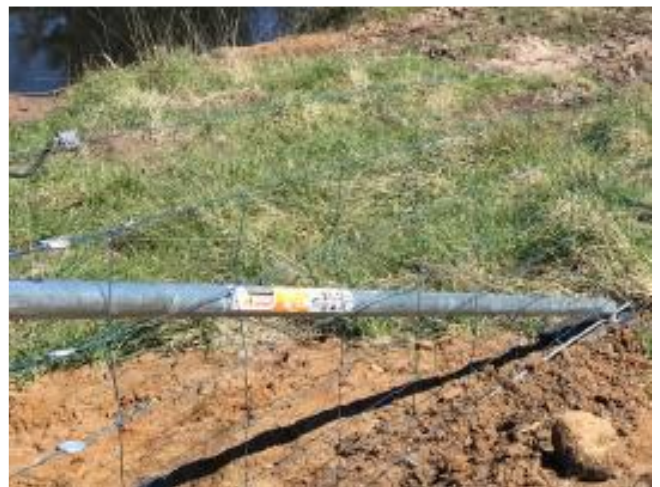
Gripples create weak sections for sacrificial sections
