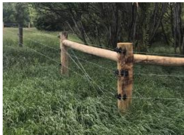
Larger end assembly posts, driven 1 metre into the ground provide increased fence resistance.
