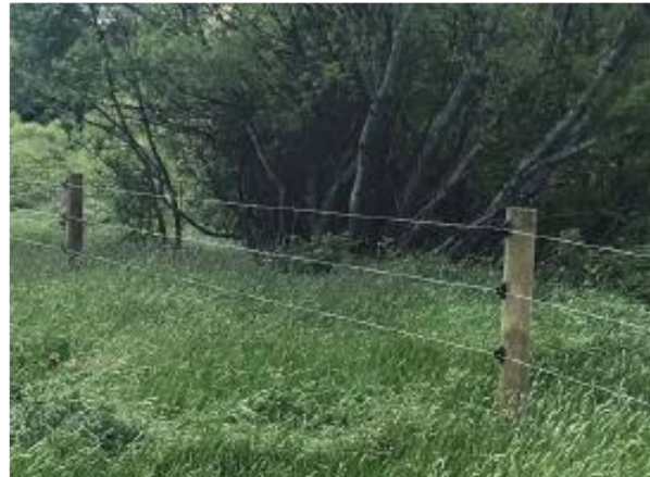
Positioning wires on the downstream side of posts means staples and insulator clips can give way if necessary.
