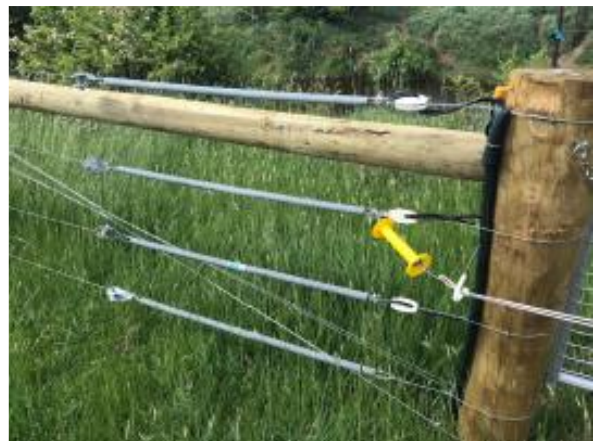
Springs at the end assemblies increase wire flexibility
