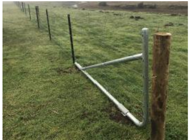
A drop fence end assembly is designed to lay flat on the ground when needed
